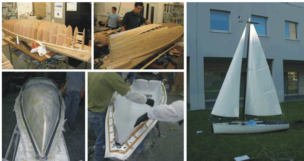
Figure 1: The construction of FAST: (top-left to bottom-right) assembly of the frames; strip planking; the mould; filling the mould with the layers of fibre and core materials; the final boat.
